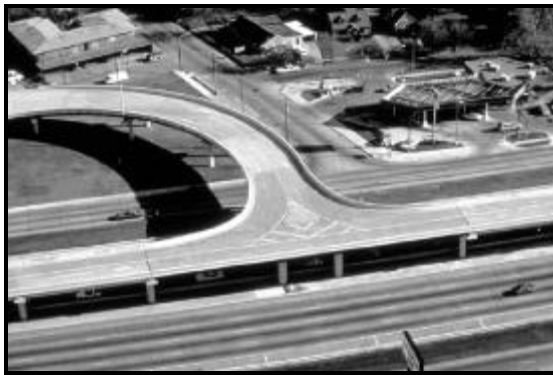
Figure 6-28. Houston Grade Separated HOV Lane Access Ramps. (9)
