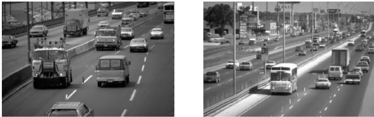
Figure 6-6. Examples of Contraflow Lanes. (9)
