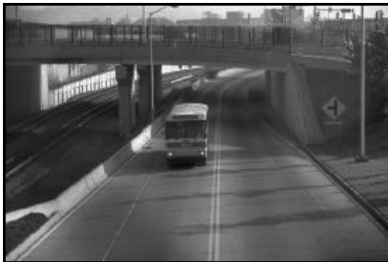
Figure 6-3. Examples of Exclusive HOV Facility - Separate Right-of-Way. (9)
