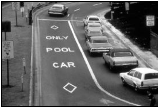
Figure 6-20. Two-Lane Entrance Ramp with HOV Bypass. (9)
