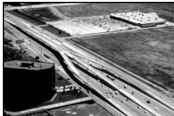
Figure 6-13. Elevated Slip Ramp. (9)
