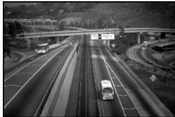
Figure 6-3. Examples of Exclusive HOV Facility - Separate Right-of-Way. (9)
