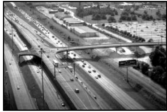
Figure 6-15. Grade Separated Interchange. (9)
