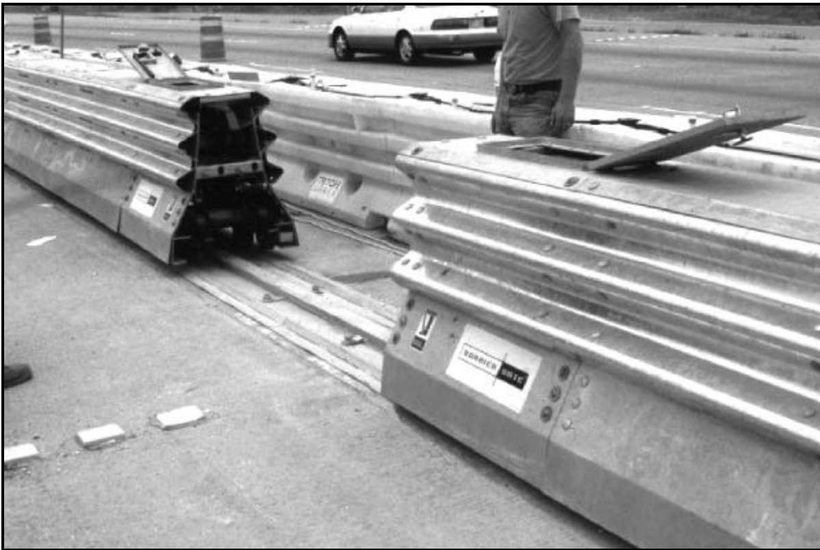
Figure 8-7. Example of Crash Worthy Barrier Gate.
